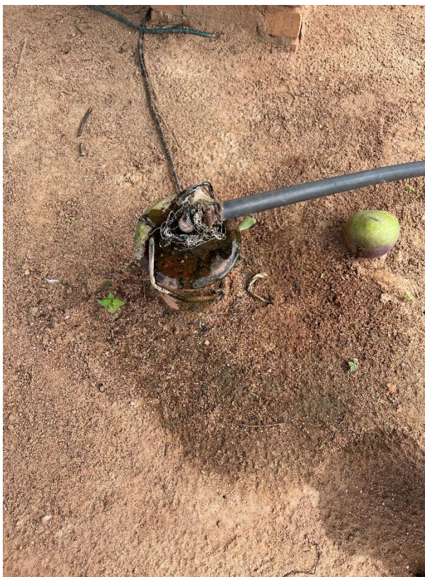
Photograph 6 – AC-06 (Private Borehole In use)
