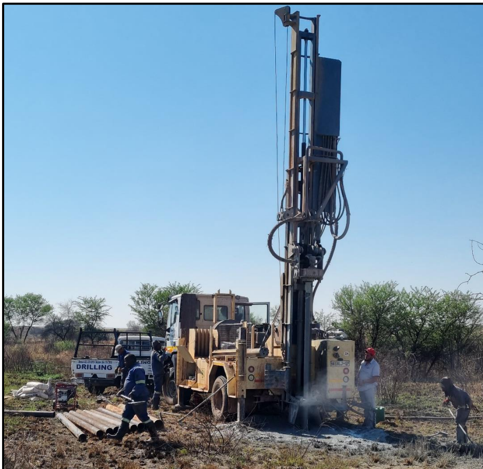
PHOTO 1: DRILLING OF MONITORING BOREHOLE
