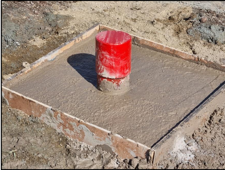
PHOTO 2: CONCRET PLINTH AND LOCKABLE CAP INSTALLED ON BOREHOLE
