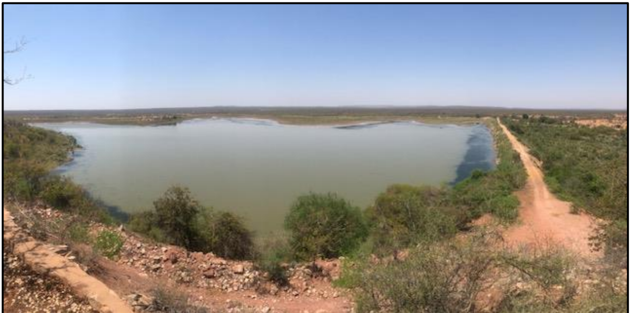
Figure 5-3. View over Lizzulea dam from the hill.
