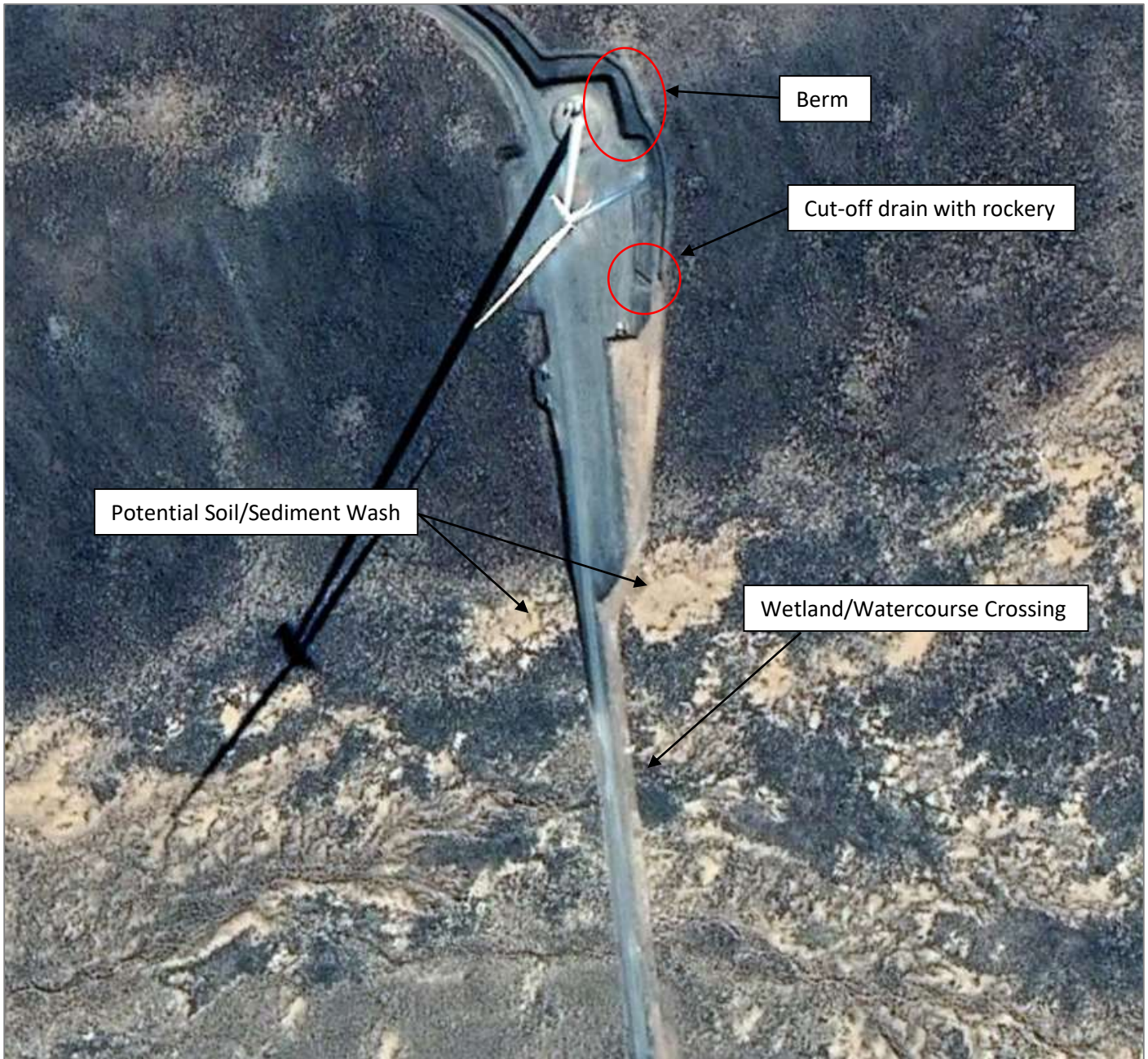
Figure 12 Existing lay-down area and turbine for the nearby Perdekraal site
