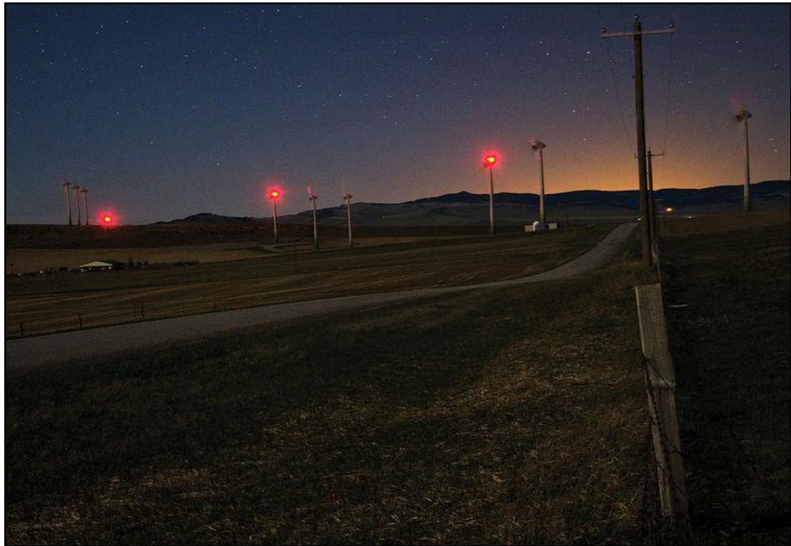
Figure 7: Aircraft warning lights fitted to the wind turbine hubs (Source: http://www.pinchercreekecho.com/2015/04/29/md-of-pincher-creek-takes-on-wind-turbine-lights. )
