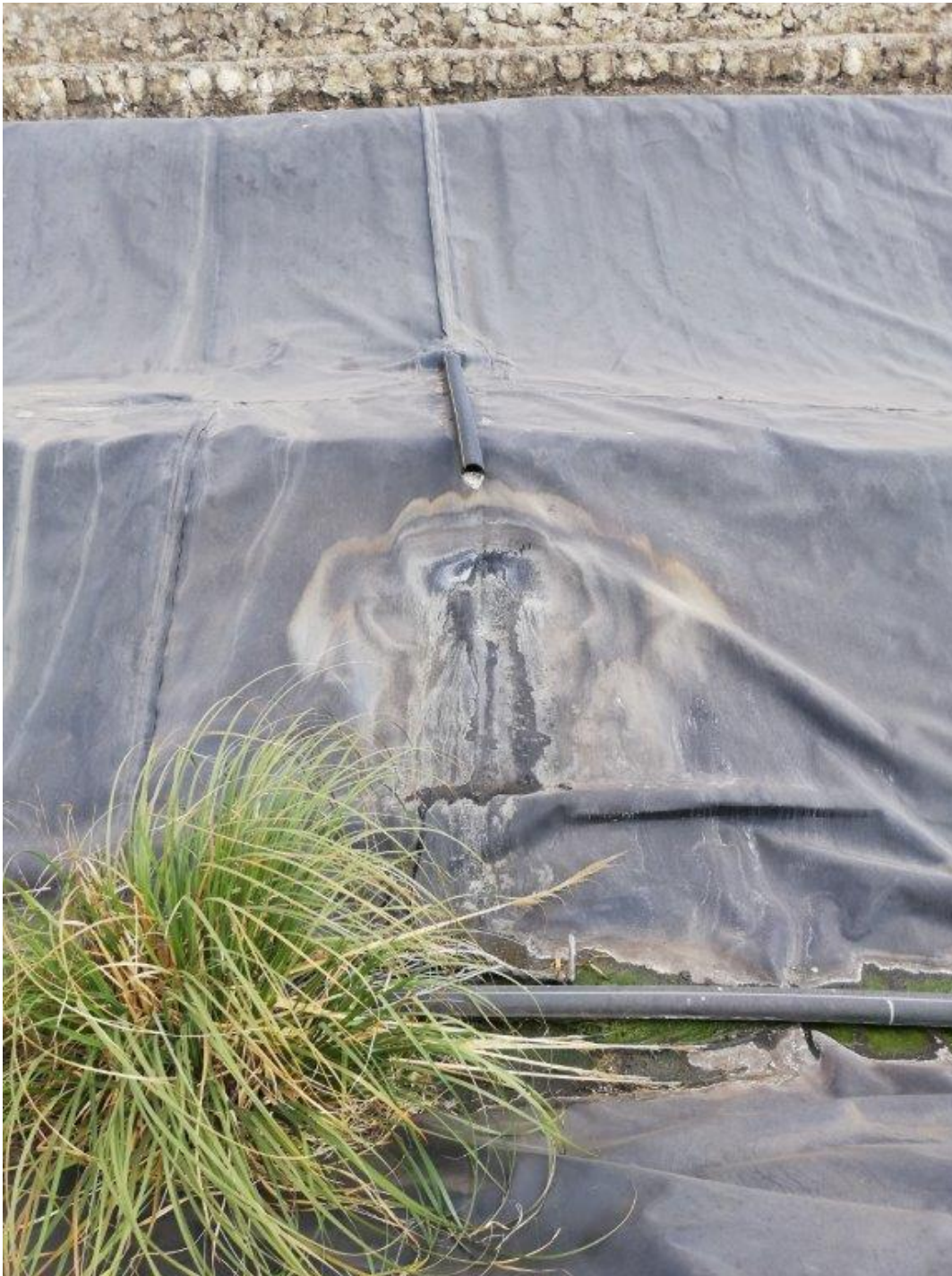
Figure 6: Tailings underdrainage pipes
