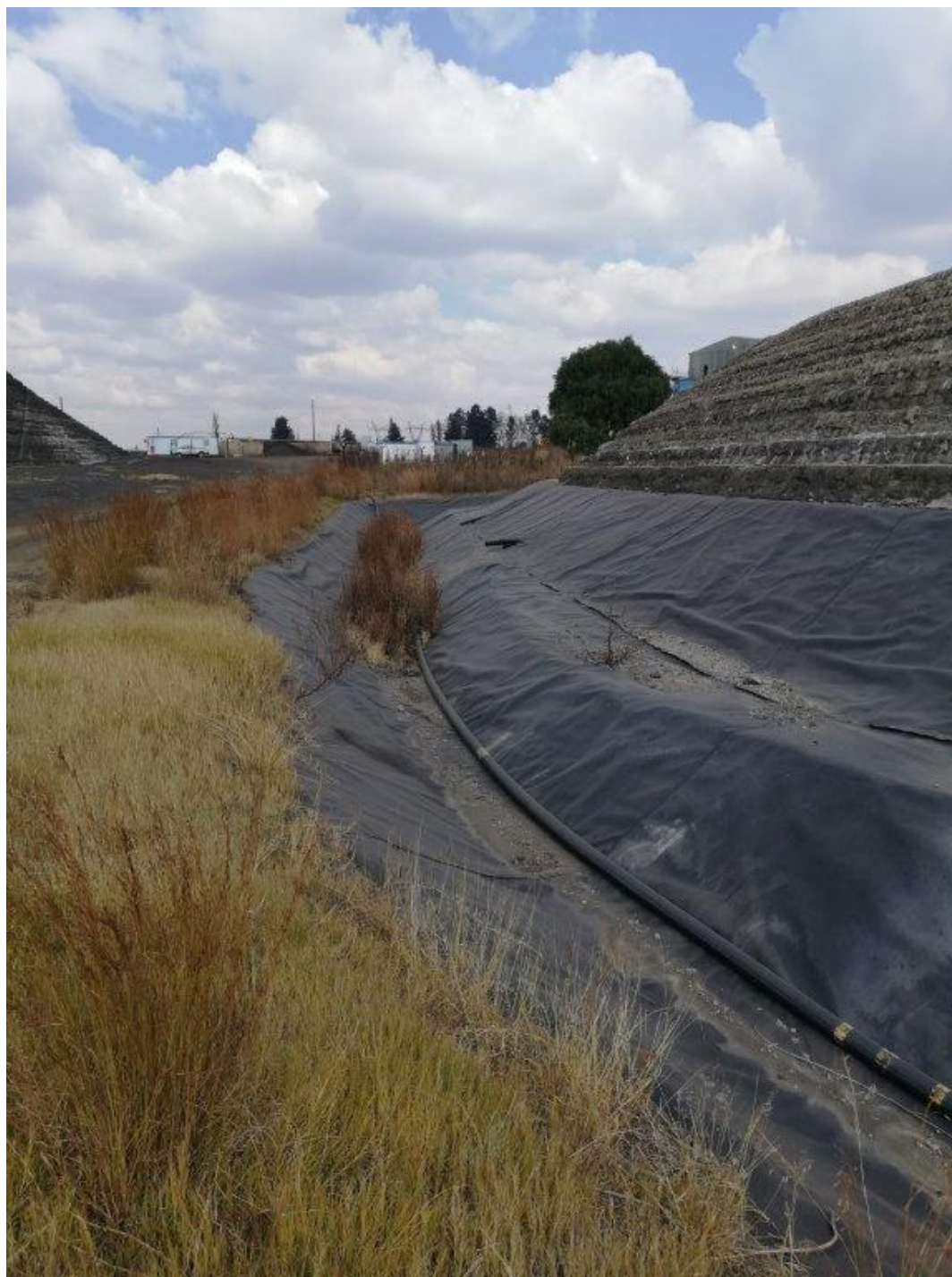
Figure 3: HDPE Liner installed in Channel and over starter wall - East wall
