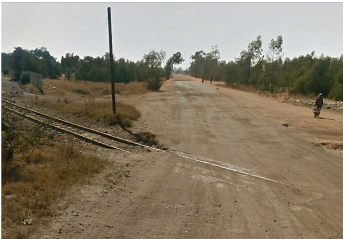
Figure 4-7: Railway tracks at main gravel road
