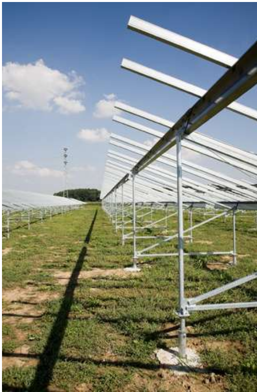
Figure 11. PV plant construction.
