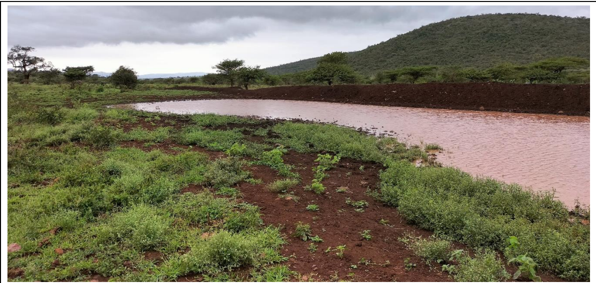
Artificial dam, collecting rainwater runoff and being used for cattle watering
