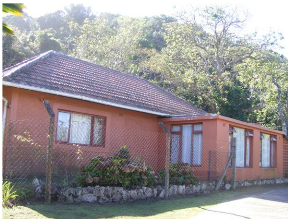
Figs 15&16: Dwelling to the north: much altered, originally thatched but reroofed in Marseille tiles. Rondawel has mono-pitch corrugated sheeting replace the original conical version
