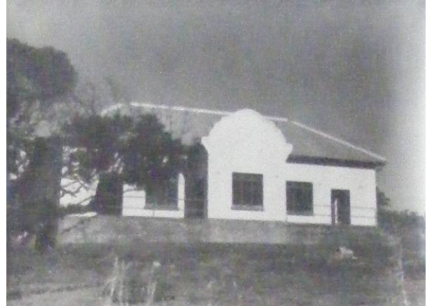
Fig 27: Old restaurant building
