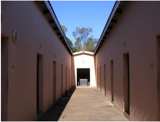
Fig 9: Open corridor, main labour quarters
