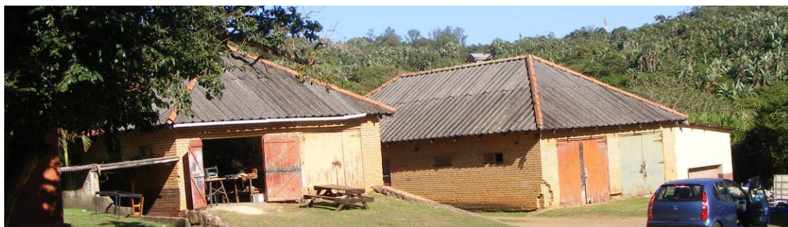
Fig 21: Utilitarian sheds to the west of the site
