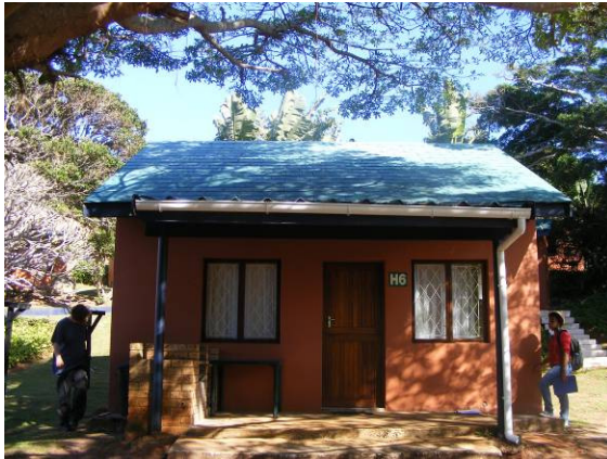
Fig 19: Older 'cottage' form
