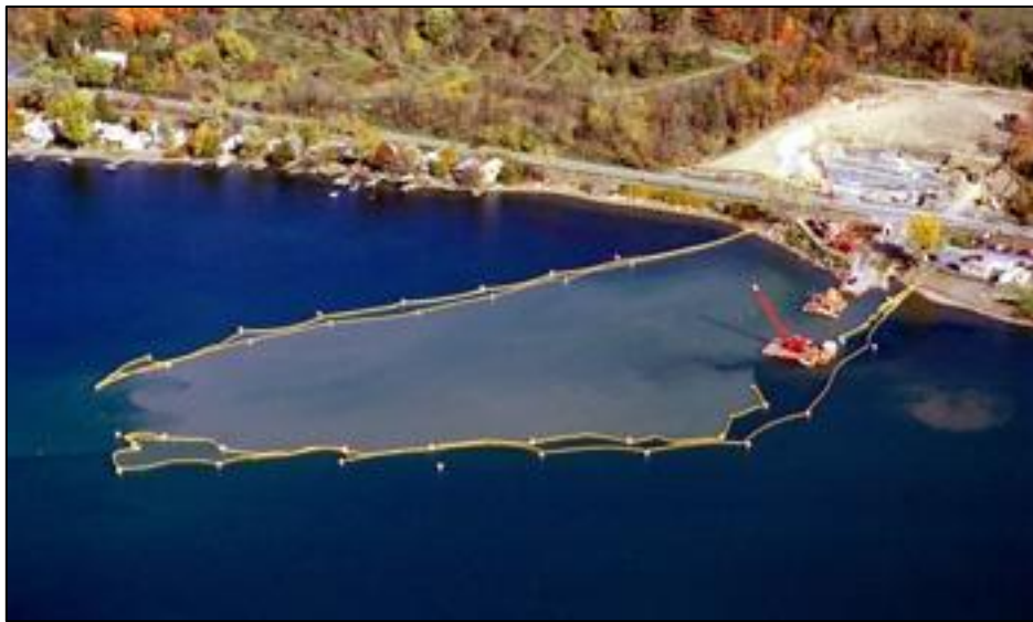
Figure 20. A silt curtain in use during construction (Source: www.landmsupplyco.com ).
