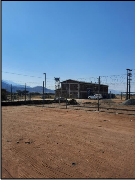
Figure 7.1. Existing Spitskop Pumpstation.
