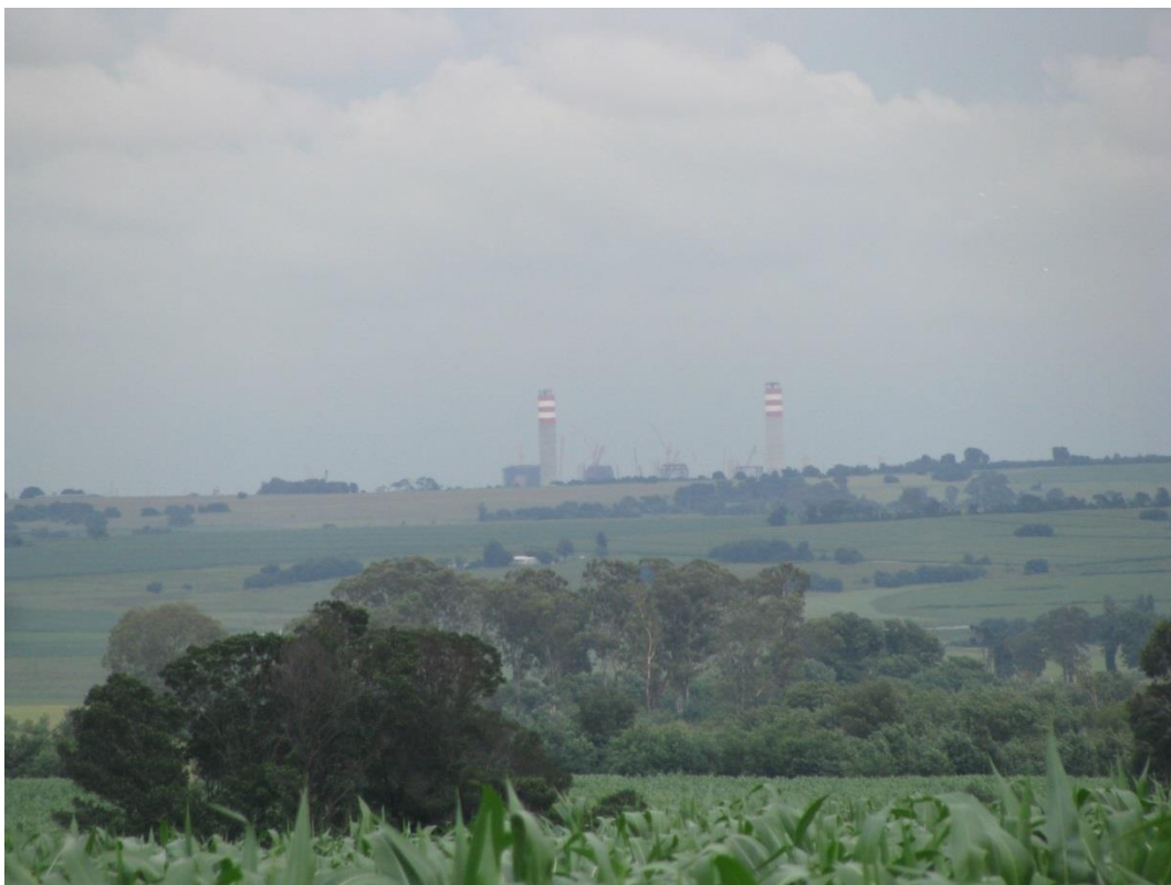
Figure 3: View of Kusile Power Station from the Project Area
