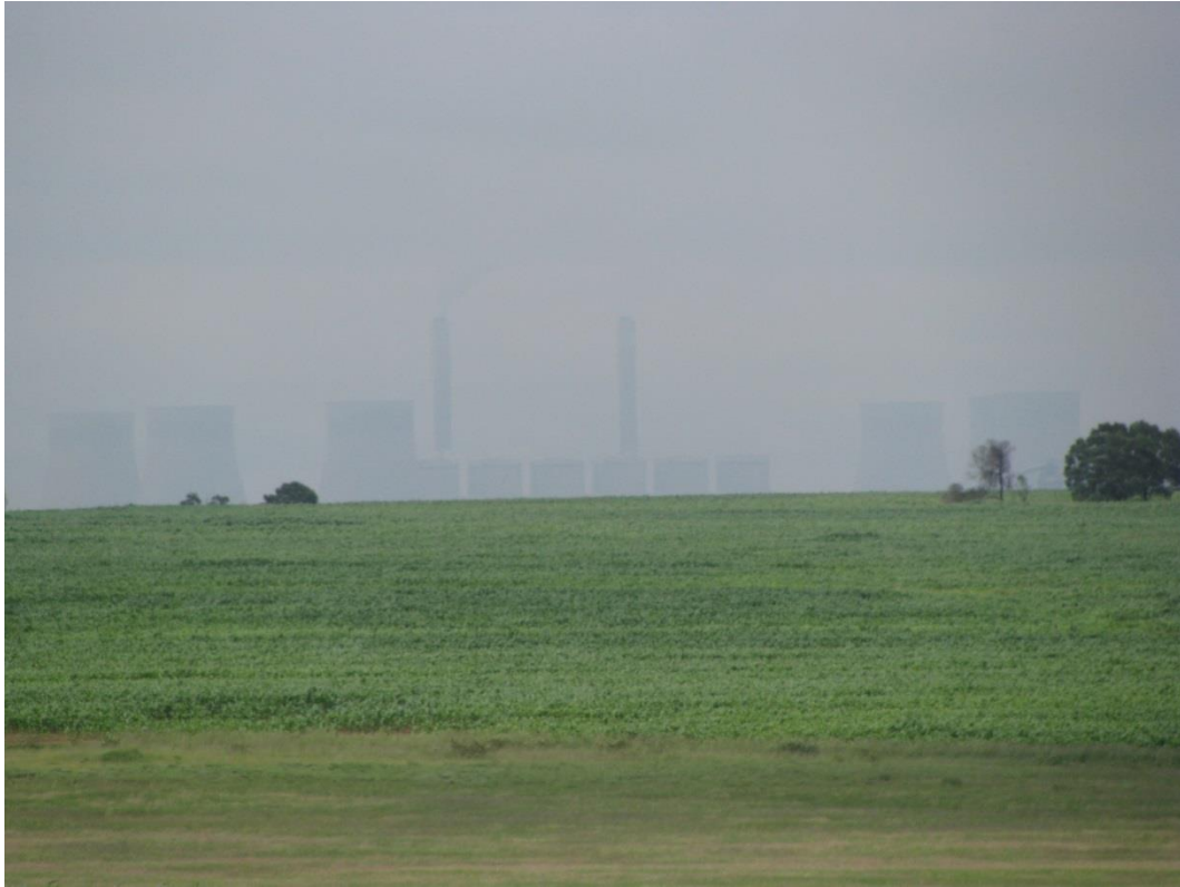
Figure 2: View of Kendal Power Station from the Project Area
