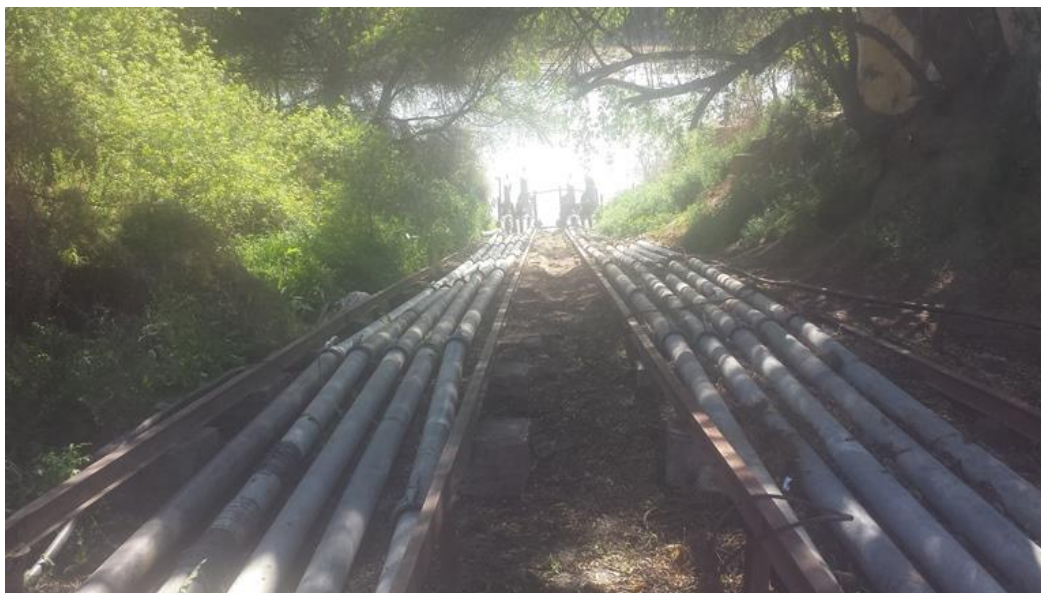
Figure 4: Existing water extraction point in the Orange River
