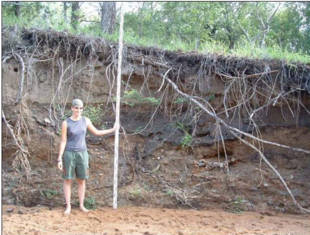
Figure 28. Eroded wall from Antonites Report (Antonites, 2005)
