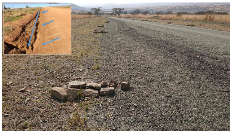
Figure 6-3 Example of road margin erosion prevention
