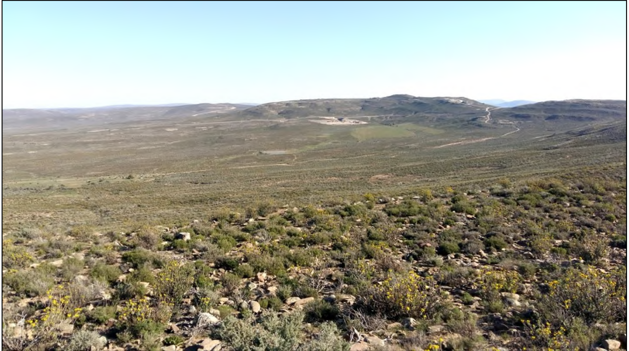
Figure 3. Looking south along the grid corridor towards the Hidden Valley substation, visible in the distance, showing the typical landscape of the affected area and the generally short stature of the Central Mountains Shale Renosterveld vegetation in the area. (Photo taken August 2020)
