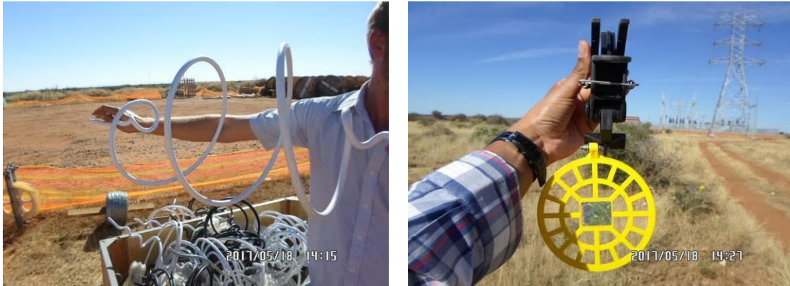
Figure 18: Examples of bird flight diverters to be used on the power lines: Double loop bird flight diverter (left) and Viper live bird flapper (right).
