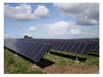
The solar facility will consist of Photovoltaic (PV) panels, which will mounted on either fixedtilt or tracking structures (to be confirmed), orientated north. Associated infrastructure will include a 132kV transmission line, an internal road network, mini-substations & transformers.
