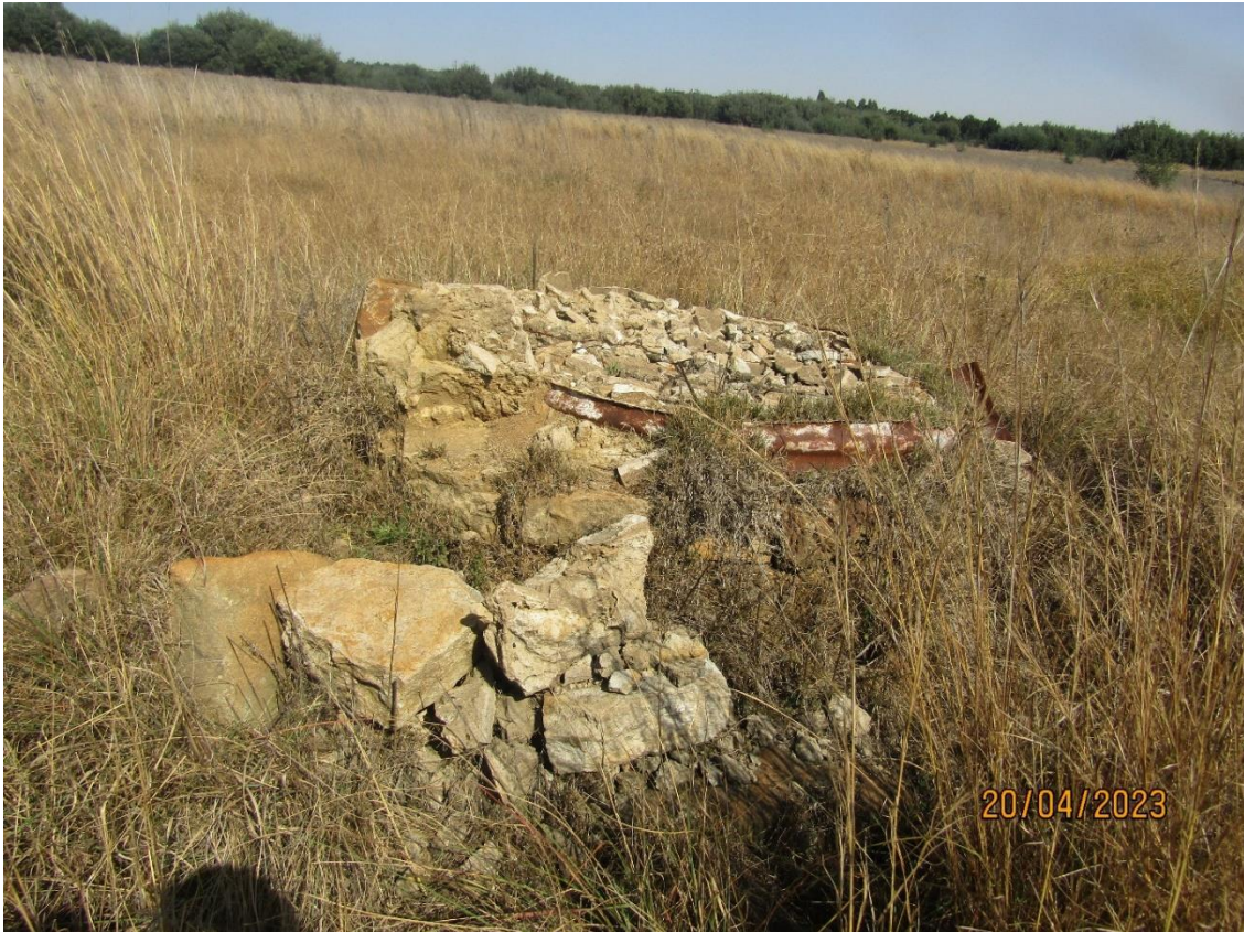
Figure 15: A wider view of the demolished old water tank as indicated in Figure 14
