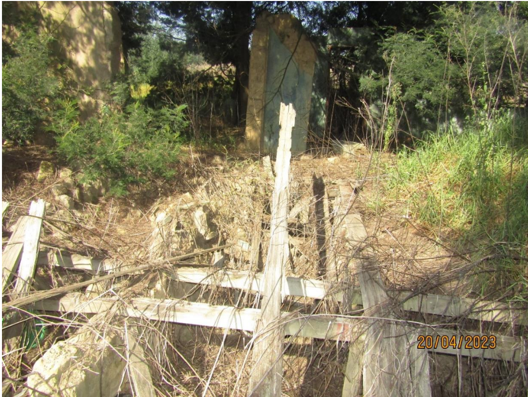
Figure 17: An old structure probably dating to the colonial times with wooden floorboards in the back ground
