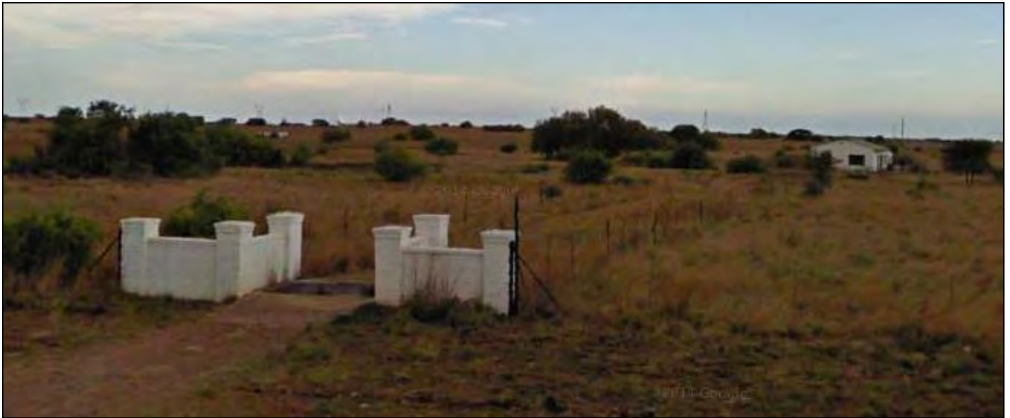
Figure 6: Eastern entrance to Houthaalboomen (PV Site) - off the R505
