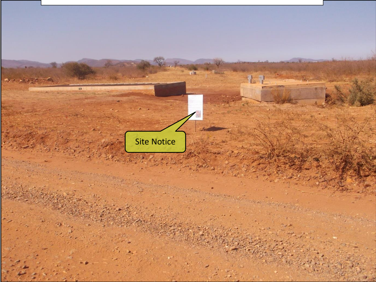
A Site Notice was placed at the end of the pipeline route at the connection point with the existing pipelines near Tshamahansi Village
