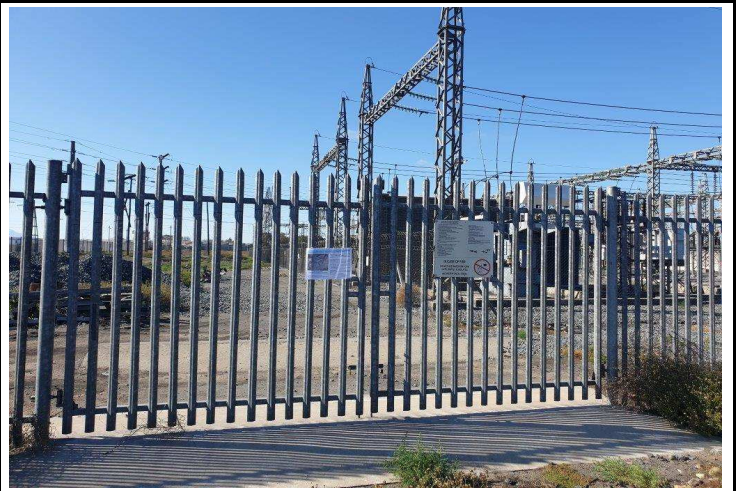
View of the notification of Public participation placed on the fence of the existing Hex Substation from the access road.
