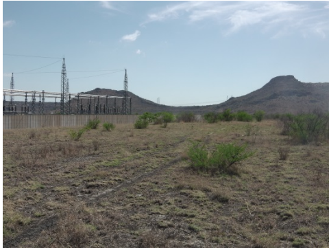
Figure 5: View towards the existing substation.
