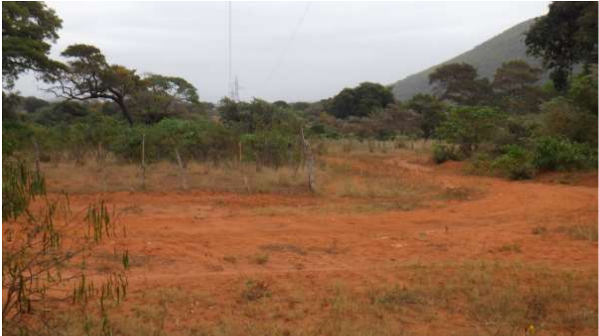
Figure 3.39: View of the T-off point (KOP Ts18) for Alternative 2. Limited screening for residents from the existing vegetation.
