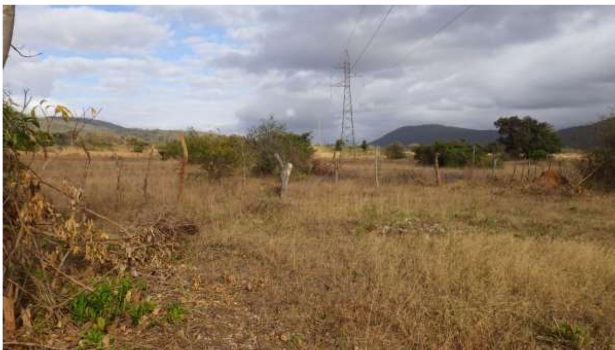
Figure 3.4: View of the T-off point from the existing power line. Cleared areas for cultivation and grazing lower the screening potential.
