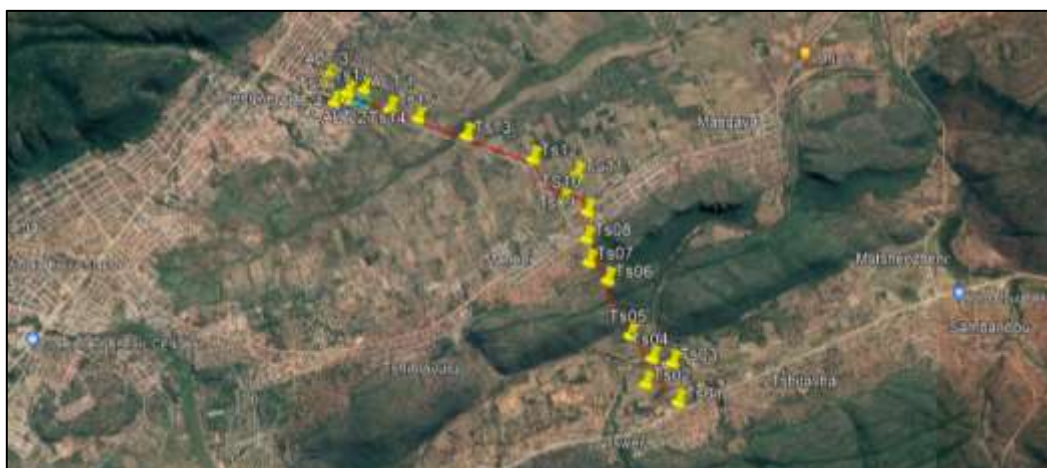
Figure 3.2: Aerial image giving a broad overview of the KOP's in relation to the larger study area.
