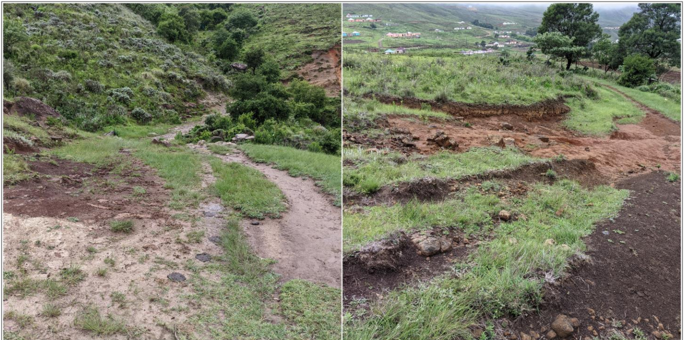
Figure 1 General site along the Sdangeni Road Extension
