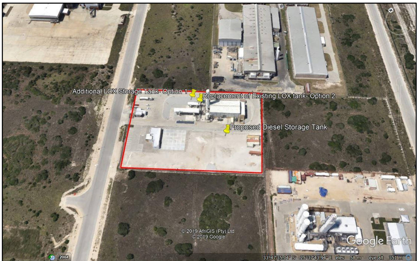
Figure 2: Proposed options of the LOX and Diesel storage alternatives on the Air Products Coega Site
