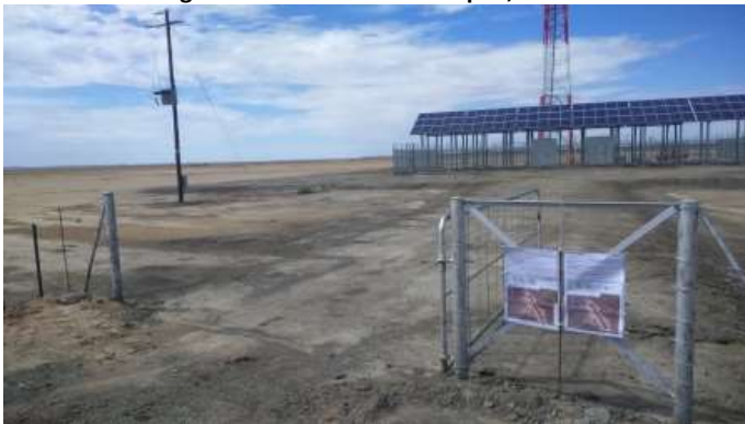
Photo 15: A2-Eng+Afr Posters at Hakskeenpan, MTN station
