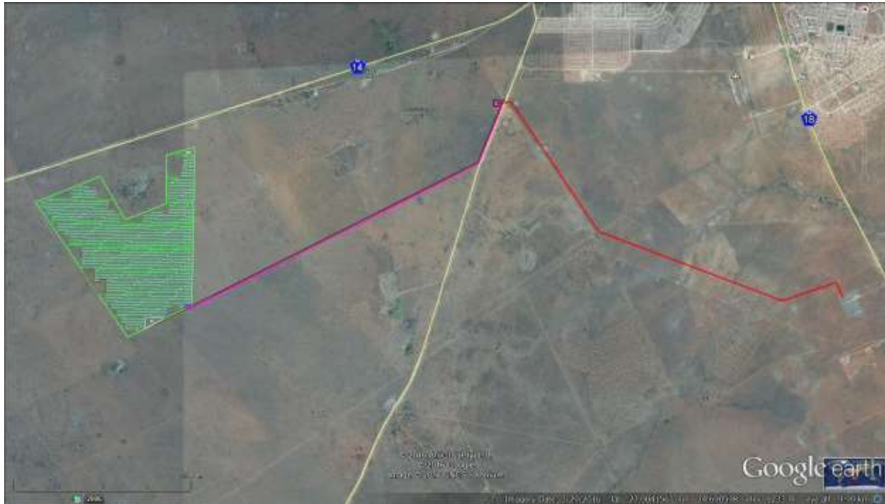
Figure 1. Satellite image of the Klondike Foxtrot site, illustrating the proposed development footprint of Klondike Foxtrot Power Plant, with the grid connection to Mookodi MTS in red.
