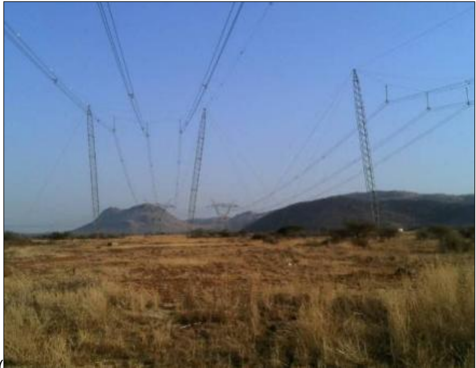
The cross rope suspension tower (
