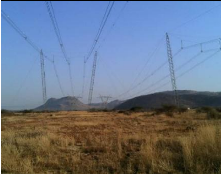
Figure 4-1: Examples of the bird friendly “cross-rop suspension” tower design
