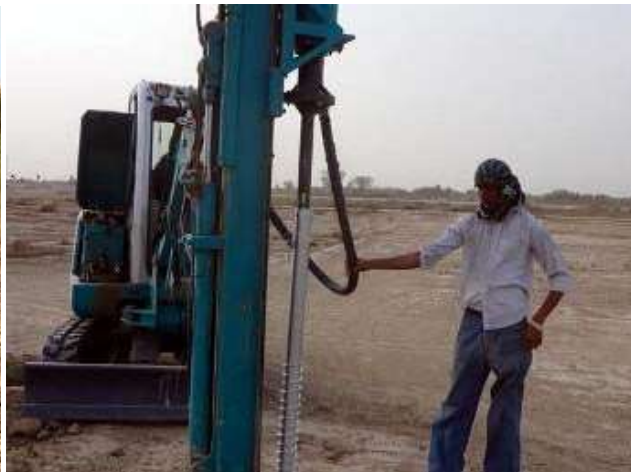
Figure 8: Ground Screw (PV MAGAZINE, 2014)
