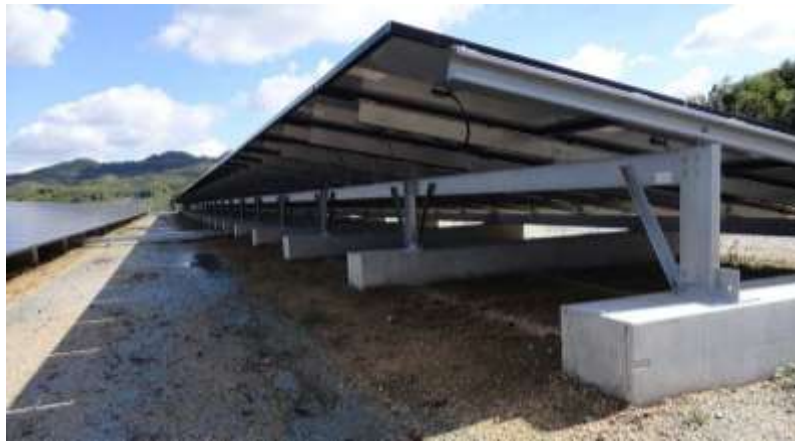
Figure 6: Cast Concrete Foundation (Solar Power Plant Business, 2013)
