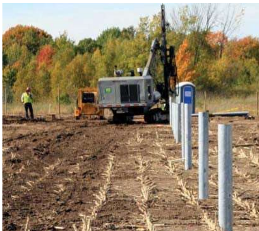
Figure 7: Driven/Rammed Steel Pile (SolarPro, 2010)
