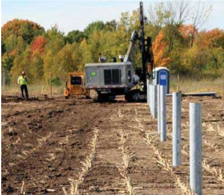
Figure 3: Rammed/ Driven Steel Pile (SolarPro, 2010)
