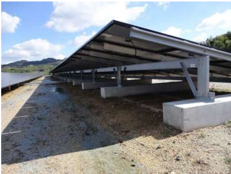
Figure 2: Cast Concrete Foundation (Solar Power Plant Business, 2013)
