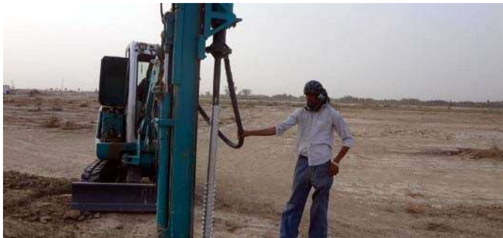
Figure 4: Ground Screw (PV MAGAZINE, 2014)
