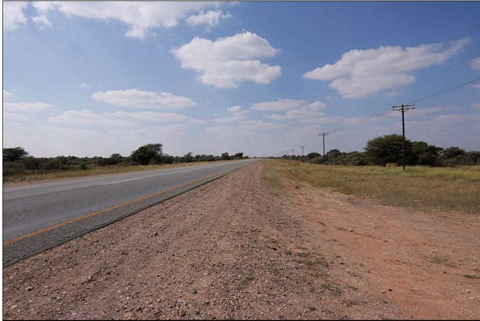
Photo 5: Sight distance to the east
