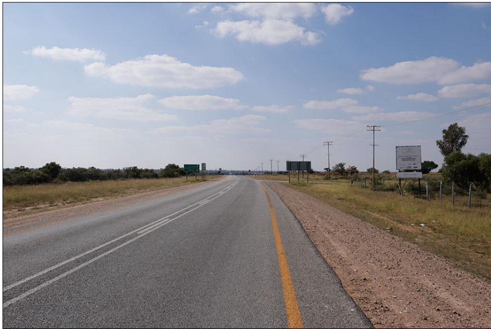
Photo 12: Good condition of N14
