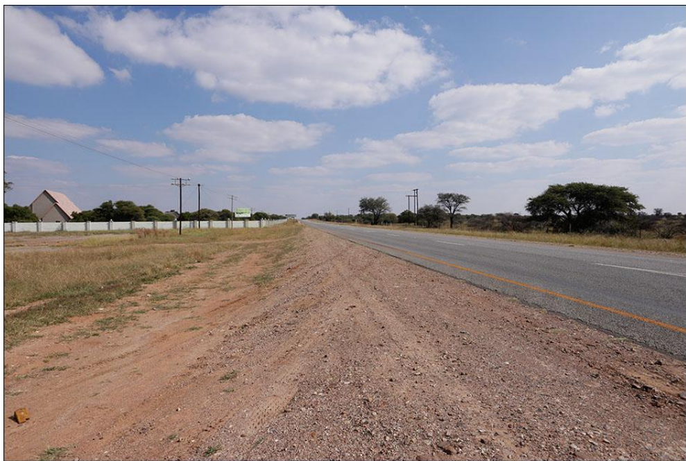
Photo 6: Sight distance to the west
