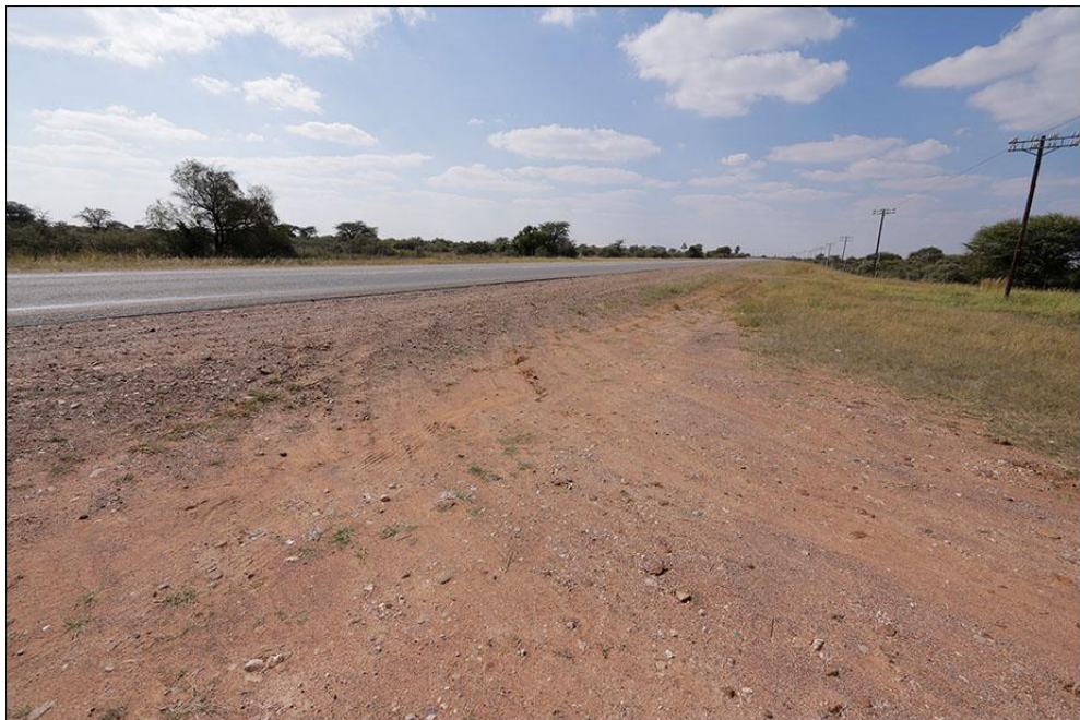
Photo 7: Gradient of access road
