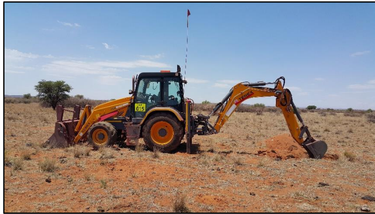
PHOTO 1: TLB USED TO EXCAVATE TRIAL PITS
