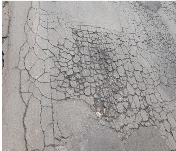
Photograph 3.4: Crocodile cracks in the pavement
