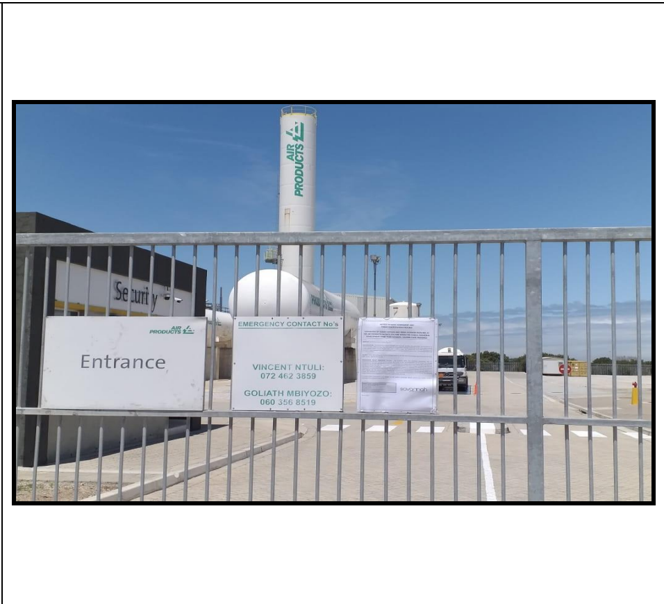
Figure 2: Site Notice (No.1) Placed at the entrance to the Air Products Coega site
