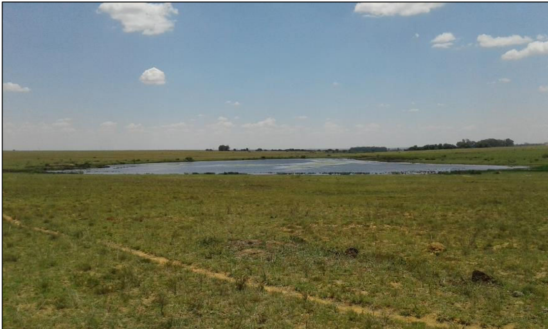
Figure 10: A large man-made dam situated at the confluence of three tributaries along the course of the un-named non-perennial drainage line north of the Kromspruit.
