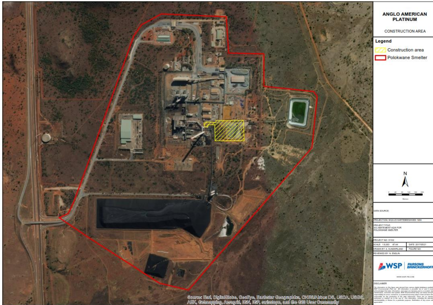
Figure 6-1: Proposed construction area at Polokwane Smelter.
