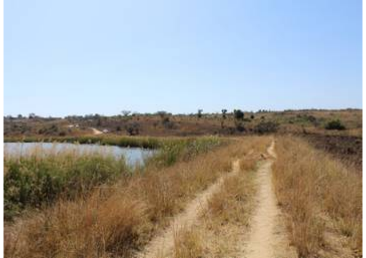
Photo 2: Dam crest (access road on dam wall)
