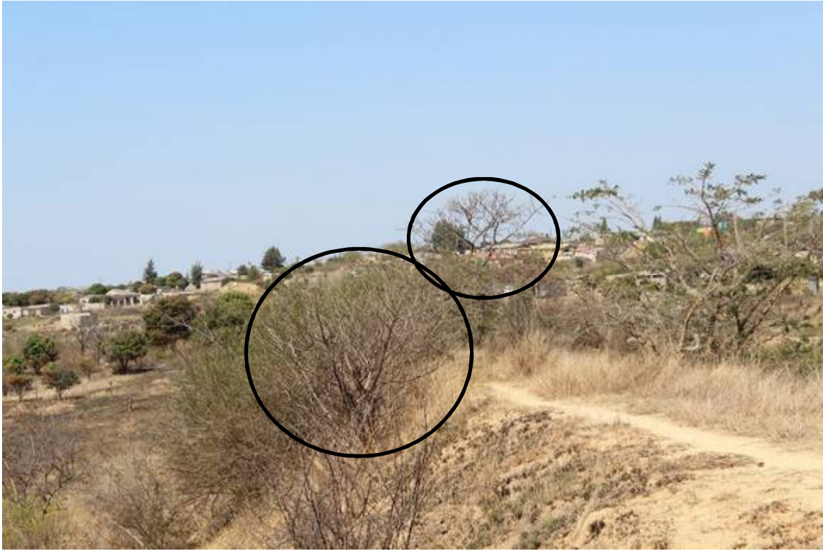
Photo 7: Several Marula trees (encircled), without leaves, located on the groin of the dam embankment.
