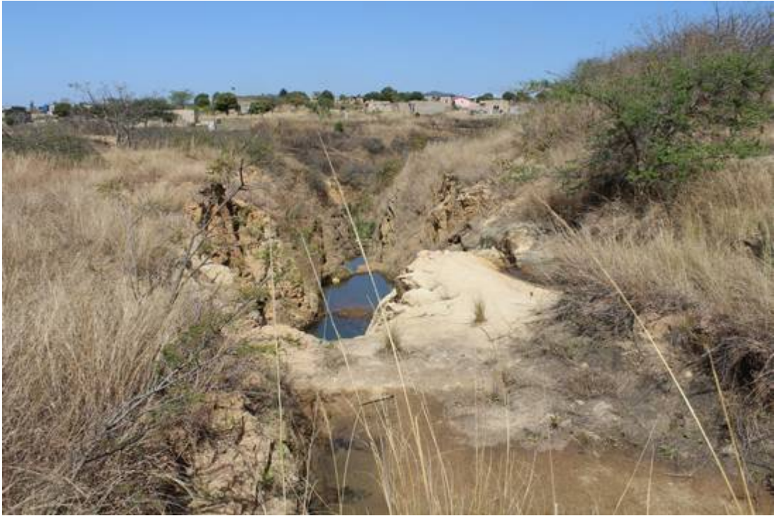
Photo 13: Large donga formed below the spillway channel.
