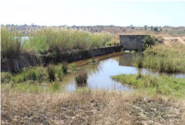
Photo 11: Sharp crested weir spillway
