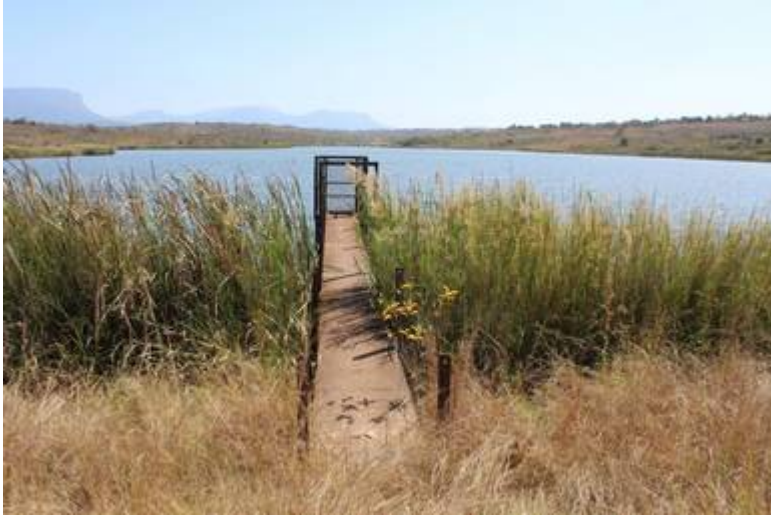
Photo 1: Casteel Dam facing upstream
