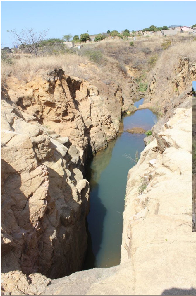
Photo 14 (left) and 15 (above): Large donga below the spillway channel.
