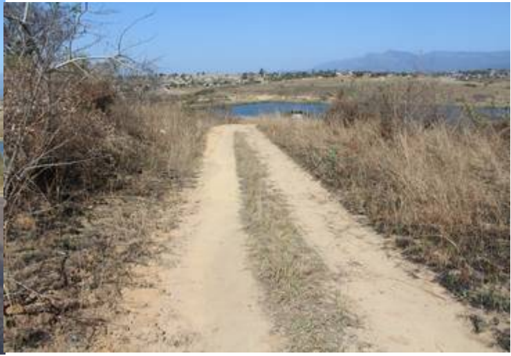
Photo 25: Existing gravel access road to the Casteel Dam embankment which will be upgraded (Section 1).
