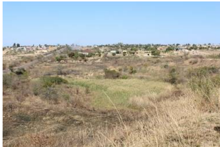
Photo 6: CVB wetland below dam embankment
