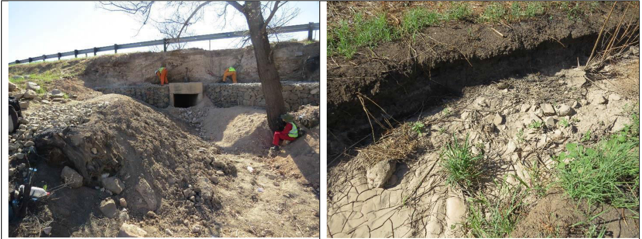
Figure 9: Impacts associated with the watercourses include invasive species and small-scale erosion of watercourses at road crossings.
