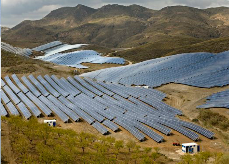
Illustration of a photovoltaic solar energy facility (Spain) (sourced from http://australianmuseum.net.au/image/Solar-Power-Plant/ )
