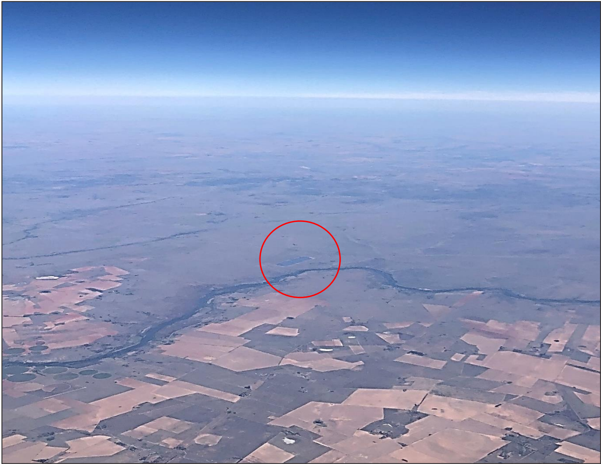
Figure 4.4: View of the Bokamoso SEF from an airplane at a height of 36000 feet amsl.
