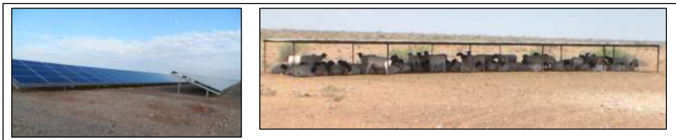
Figure 16: Ground clearance under PV panels in comparison with shelter provided to sheep.
