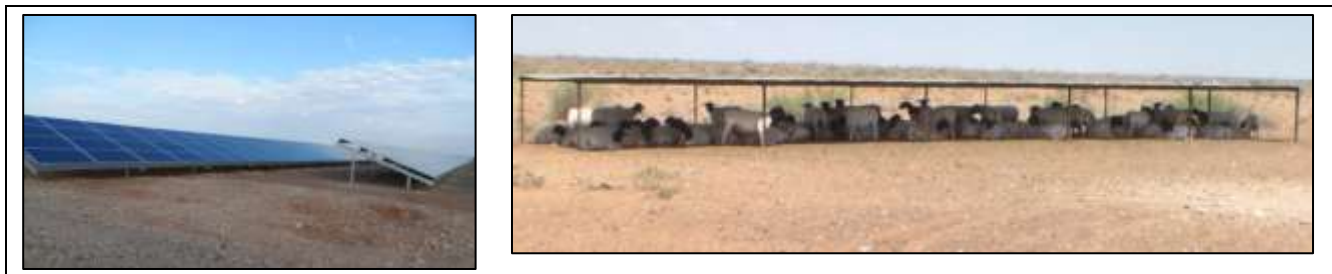
Figure 16: Ground clearance under PV panels in comparison with shelter provided to sheep.
