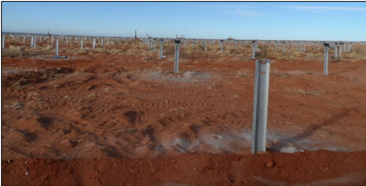
Figure 13: Status of vegetation during construction of mounting systems.
