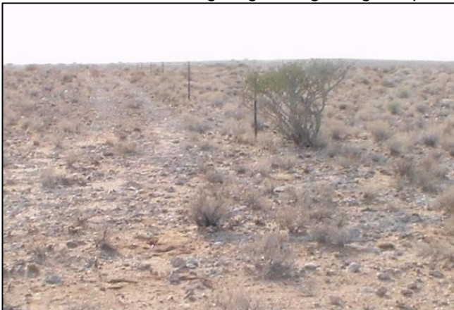
194 Fence in process of demolition. Shallow soil with surface stones
