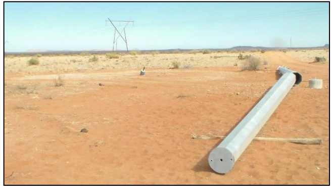
24 Shallow soil, construction transmission line
