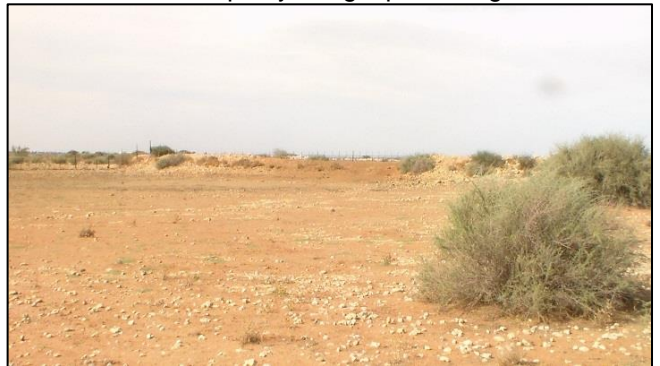
132 Earth dam, hard carbonate surface
