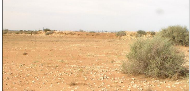
132 Earth dam, hard carbonate surface
