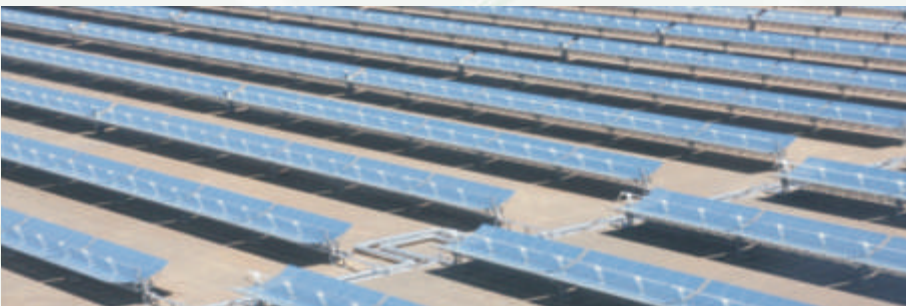
Figure 2: Parabolic Troughs
