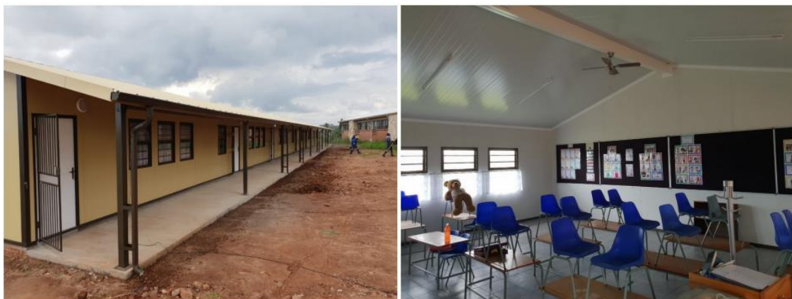
Figure 1: Typical examples of pre-fabricated classrooms
