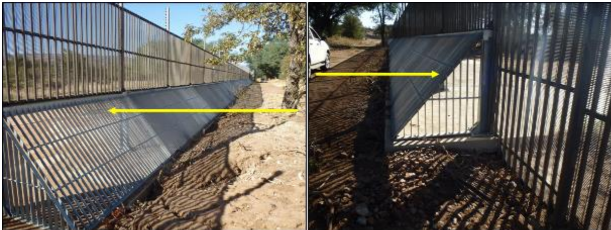
Figure 15: A grid and concrete base forms part of the study area boundary fence which crosses the Mutamba River. The yellow arrow indicates the direction of flow.
