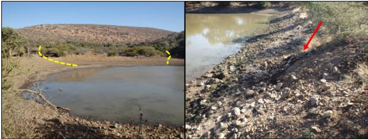
Figure 24: (Left) the EDLs (yellow dashed lines) upstream of Dam 2; (right) the red arrow indicates the pipe releasing water into Dam 2.
