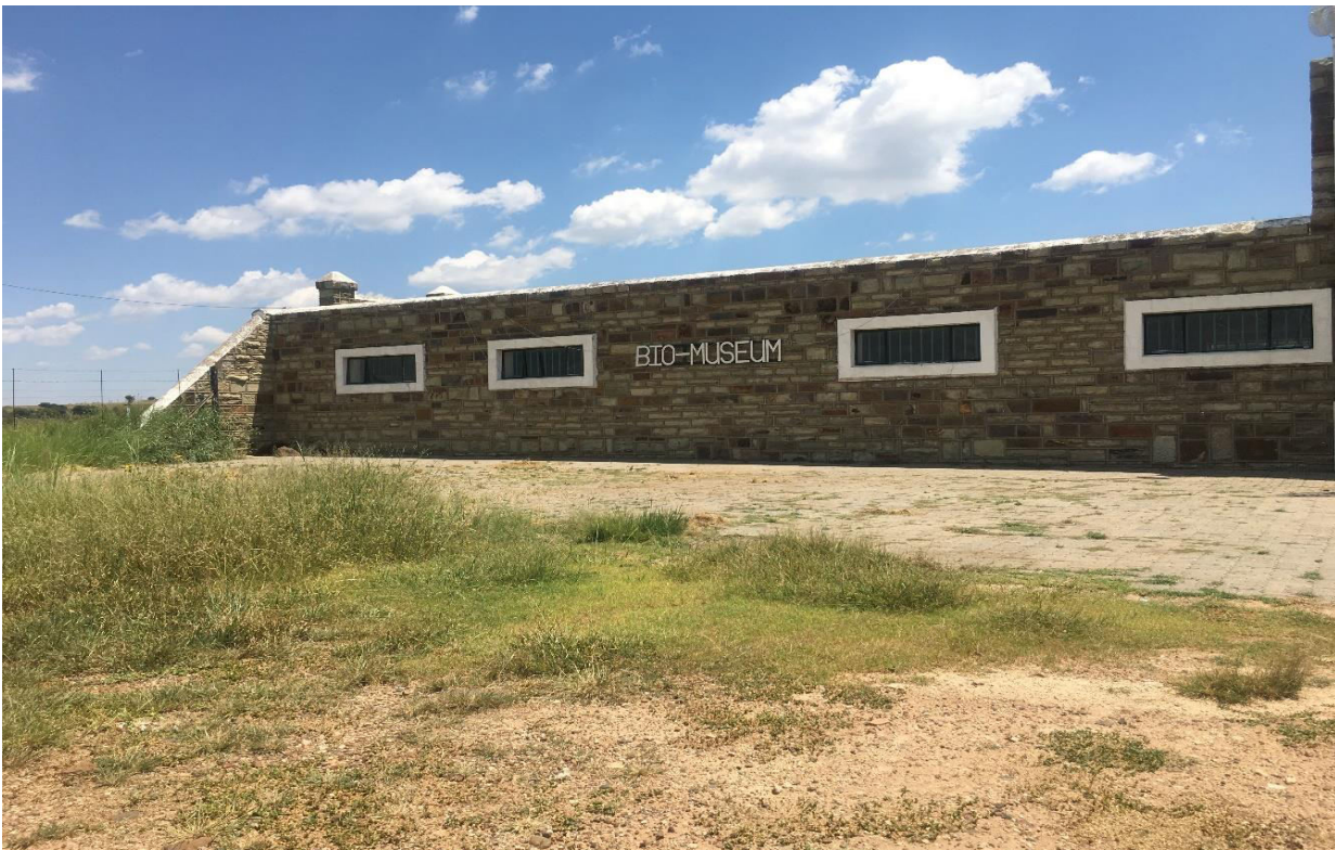
Figure 3: View of the Museum structure.
