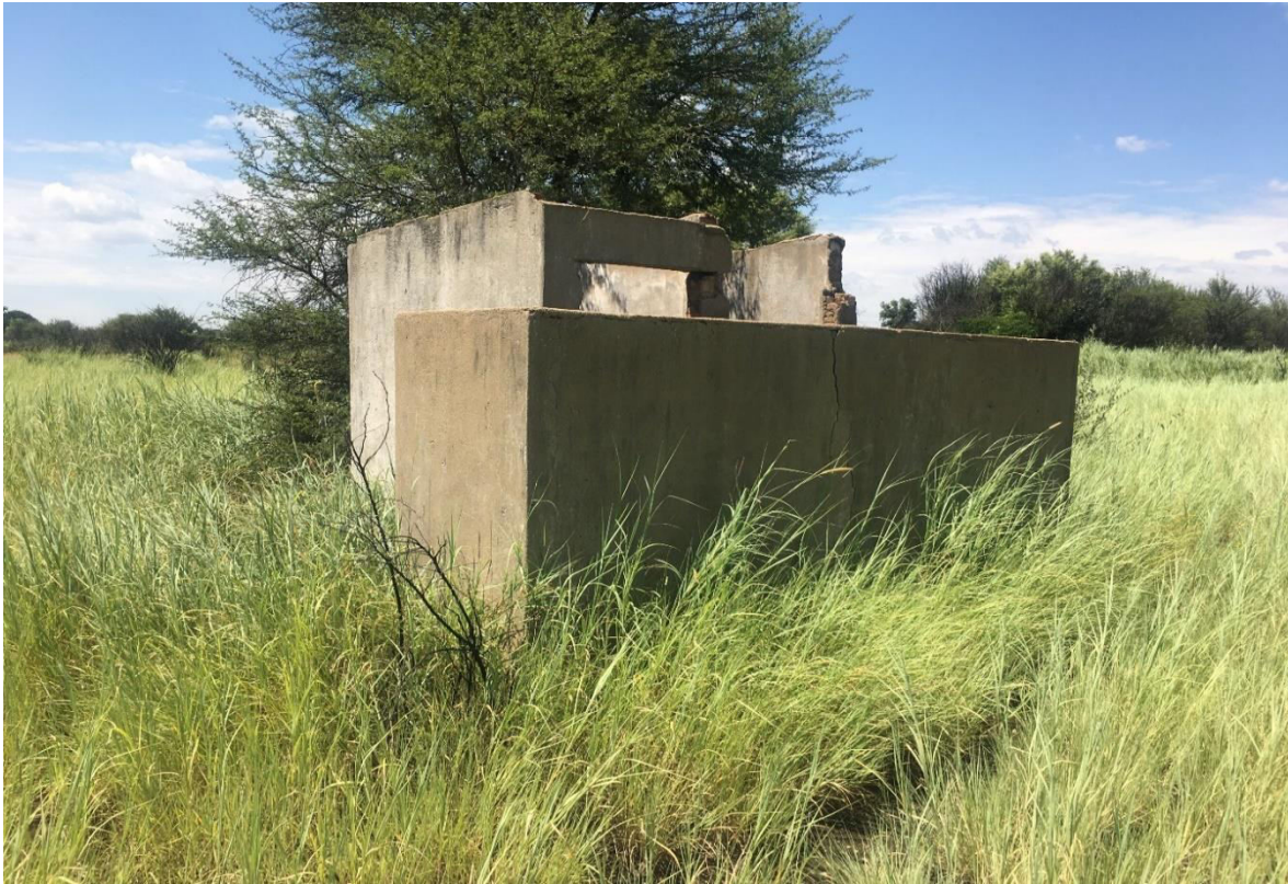
Figure 14: Structure noted on the proposed area.
